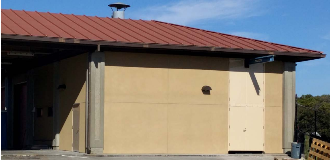
Maintenance Building Enclosed Bay
