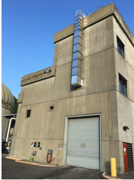
New ducting on SHB Exterior
